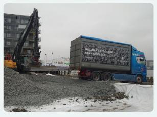
The groundwork for an extensive and challenging construction project was solved with foam glass.
