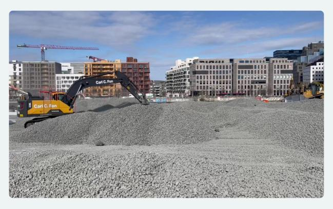
30 000 cubic metres of Glasopor foam glass aggregate were installed to prepare and level the ground in the park area.
